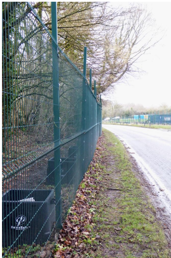
West side, showing footpath now behind the security fence, and the narrow gap remaining for pedestrians
